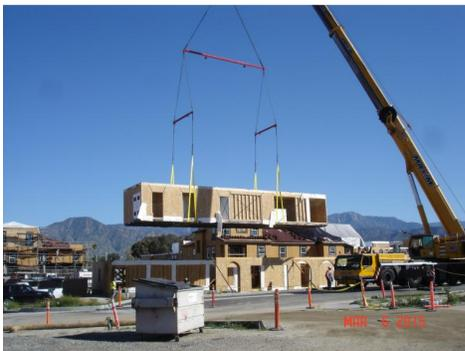
The modular construction, a first for HACSB and HPI, is a hybrid construction process, wherein the building exterior envelope and all interior finishes were completed at the Silver Creek Industries factory, then transported to the site and set by crane. Once in place, Perera Construction completed all exterior finishes and added various architectural components to complete the product, making it indistinguishable from traditional site built construction.
