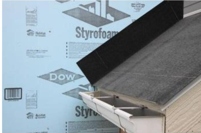
**Figure 2.** Apply roof underlayment over roof deck and up sidewall over the rigid foam insulation.
