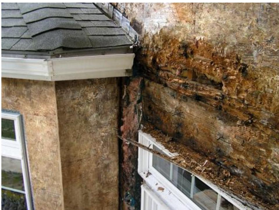
**Figure 1** - Improper flashing can allow rain water into walls, causing significant damage
