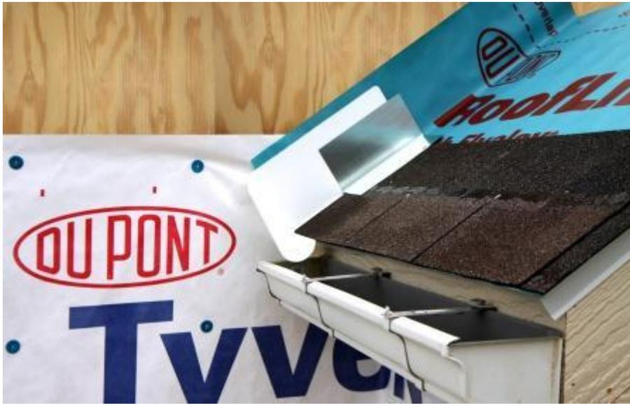
**Figure 10.** Place first shingle and next section of sidewall flashing over upper edge of diverter.
