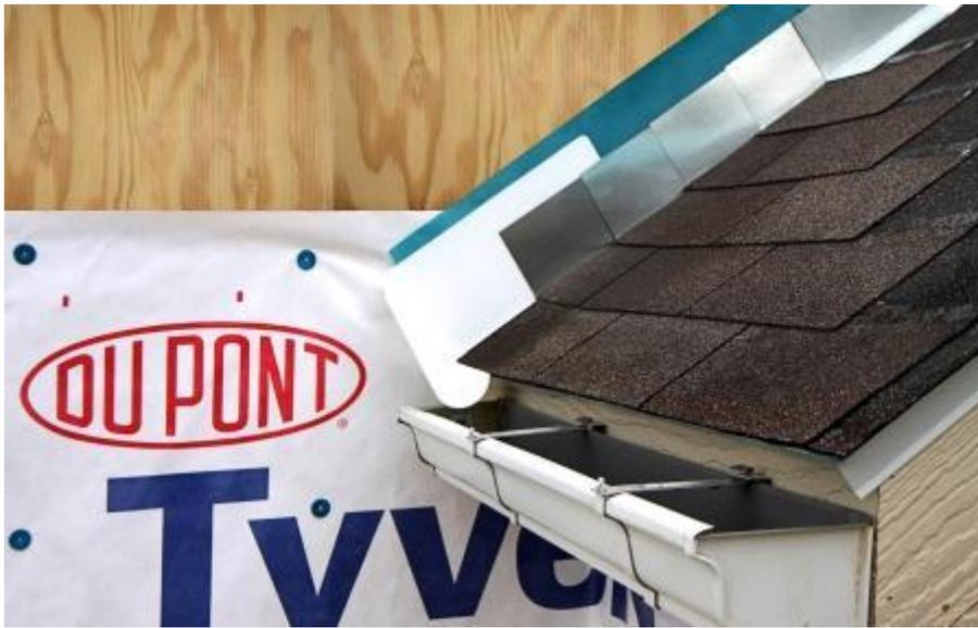
**Figure 11.** Install remaining sidewall flashing, counter flashing, and shingles.
