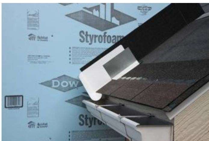
**Figure 4.** Place the first row of shingles and the first piece of flashing over the upper edge of the diverter.
