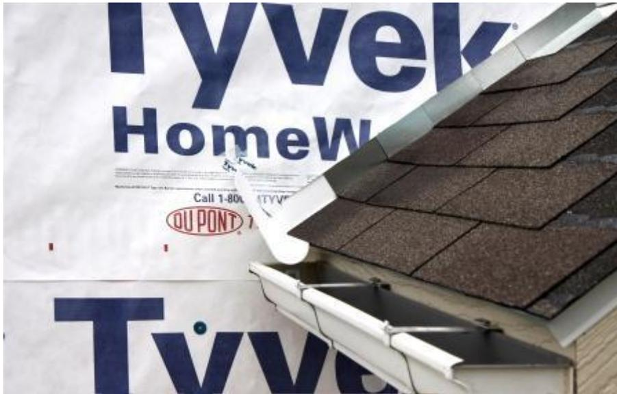
**Figure 13.** Install the housewrap. Cut housewrap to fit over diverter and tape top of cut.
