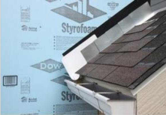
Step and kickout flashing should be installed at all roof-wall intersections to protect the wall and divert rainwater runoff into a gutter.
