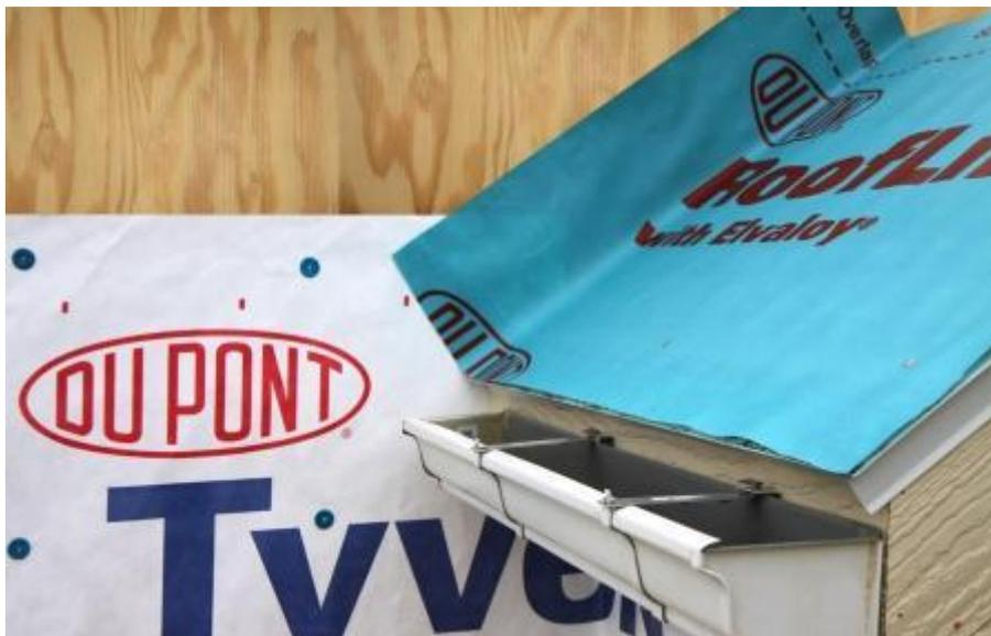
**Figure 8.** Apply roof underlayment over roof deck and up the sidewall over housewrap.
