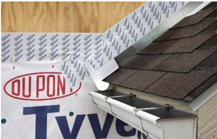
**Figure 12.** Apply self-adhesive flashing over top edge of the wall flashing, diverter, and housewrap.
