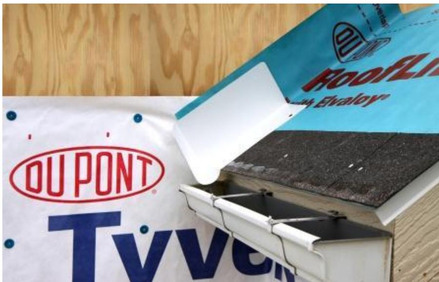
**Figure 9.** Install shingle starter strip then kick-out diverter; attach to roof deck but not sidewall.
