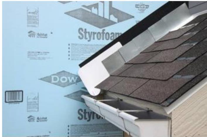
**Figure 5.** Install remaining sidewall flashing and roof shingles.
