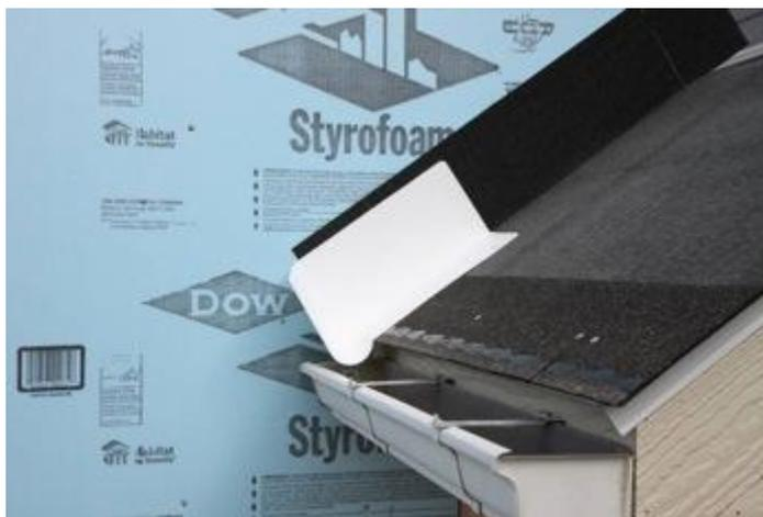
**Figure 3.** Install shingle starter strip then kick-out diverter as first piece of step flashing.
