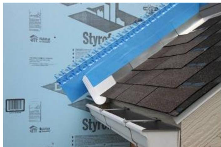
**Figure 7.** Apply construction tape over the self-adhered flashing.
