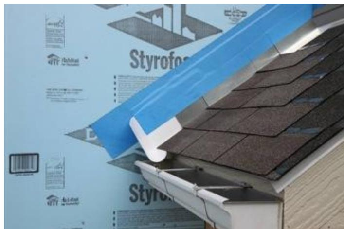
**Figure 6.** Apply self-adhesive flashing over the top edge of the wall flashing, the diverter, and the rigid foam insulation.
